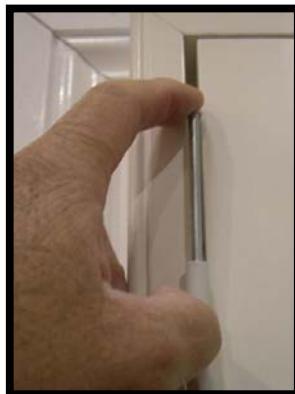
Use hinge pin to attach the panel to frame.
